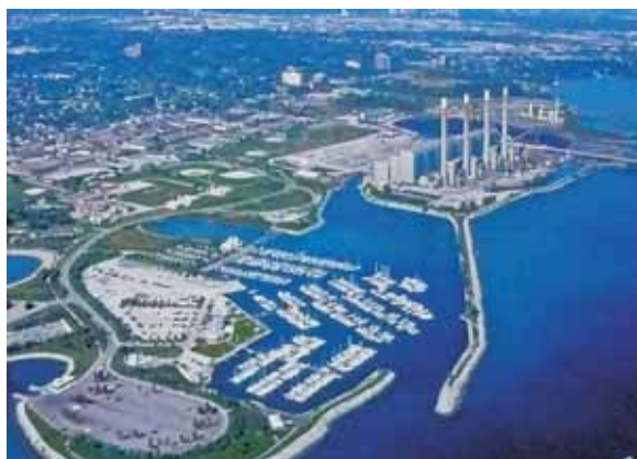
Professor John Danahy and Jim Tovey (top) looking over conceptual designs for the Lakeview lands that used to be home to a giant power plant (above). Danahy calls plans for the 500 acres a magnificent vision of a complete urban waterfront. Photos by Rich Letkeman
